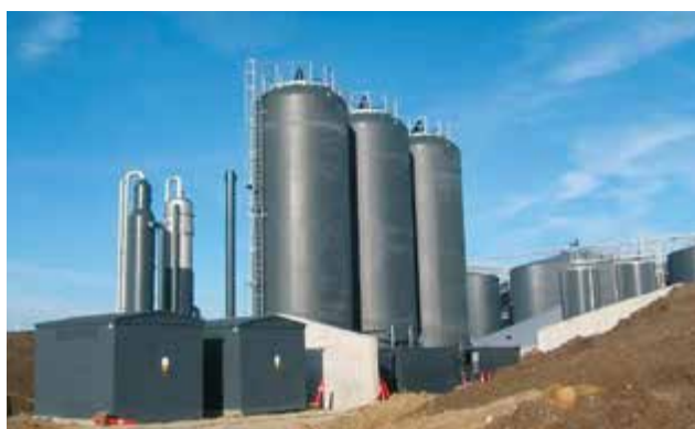
FIGURE 5.5 Biogascleaner QSR desulphurization plant to NGF Nature Energy Korskro in Denmark. PHOTO Biogasclean.
