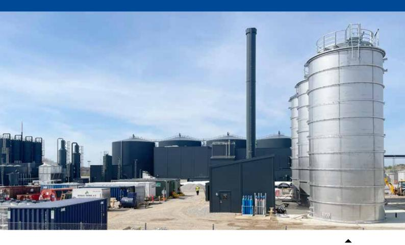
Biogasclean has developed a ground-breaking technology which converts  $CO_2$  from a harmful greenhouse gas to a sustainable green fuel. In the Bio E-Fuel reactor a biological process converts carbon dioxide ( $CO_2$ ) and hydrogen ( $H_2$ ) to methane ( $CH_4$ ). Hydrogen is made from electrolysis of water powered by wind and solar. The conversion of power to gas or liquid is called Power-To-X (P2X). A key advantage is that methane – unlike electrical power – can be stored.
