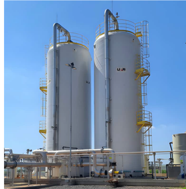
Plant: AB Brasil Pederneiras, Brazil Capacity: 1,430 m 3 /h (841 scfm) biogas 10,400 ppm H 2 S
